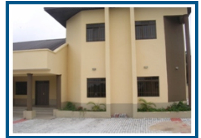
Police Clinic - One of the 165 Health Centers Constructed by the Rivers State Government
